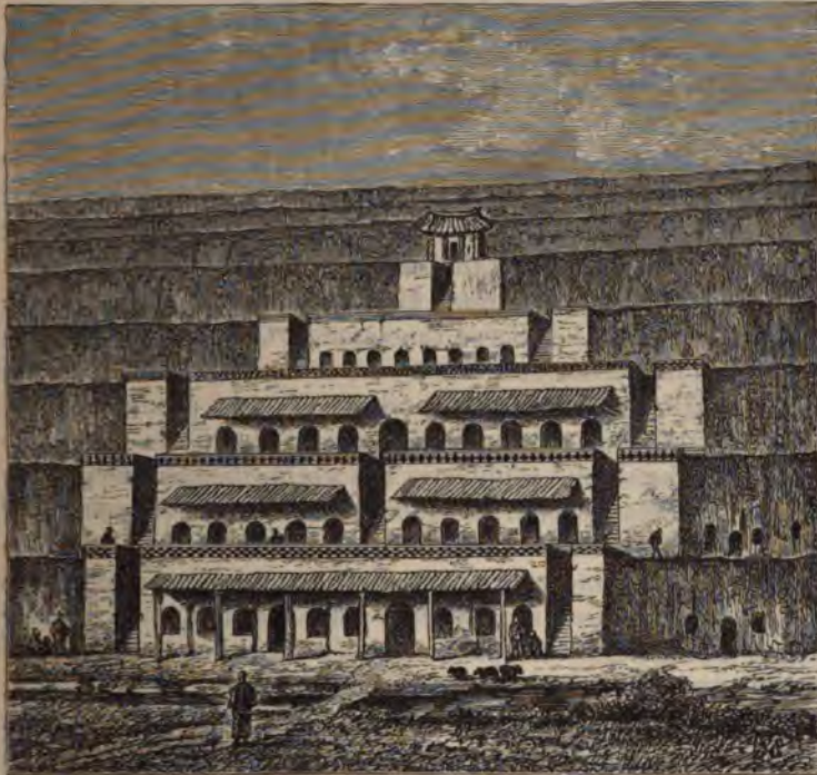
Facade of Dwelling in Loess Cliffs, Ling-shi hien. (From Richthofen.)
